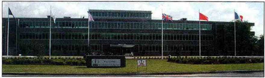
The i.park facility in Lake Success has attracted tenants looking for data recovery facilities and disaster recovery space.
