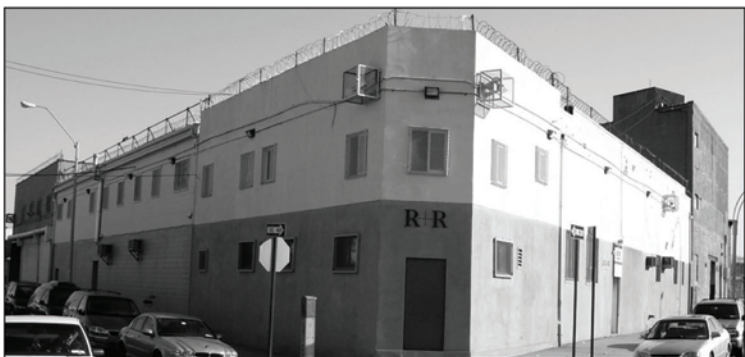
23,000 sf plus parking, centrally located with 7,000 sf of mezzanine offices and 2 interior loading platforms. For sale.
