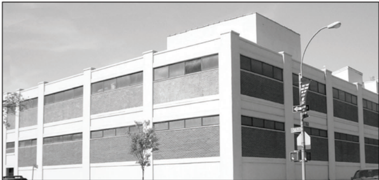
12,000 sf, fully fireproof and sprinklered loft next to Astoria Film Studios. Competitive rental.
